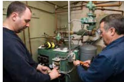
*Dave Yates, owner of York, PA-based F.W. Behler, Inc, and Technician Larry Lawrence begin disassembly of the original oil-fired New Yorker boiler at the beginning of the hydronic system retrofit.*
