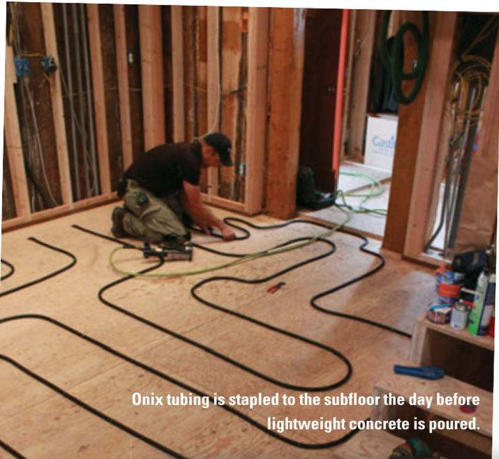
Onix tubing is stapled to the subfloor the day before lightweight concrete is poured.
