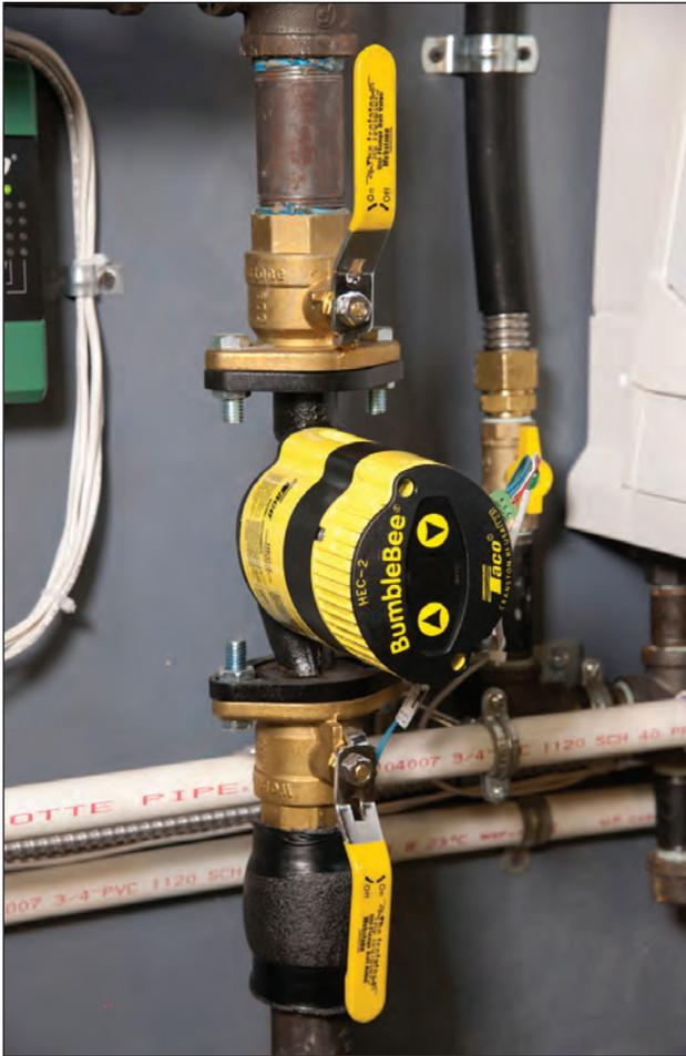
*“For high efficiency, I knew I’d point the system toward 20-degree delta-T operation, a job that would be performed by Taco’s small, bright yellow ECM circulator, the Bumble Bee,” Chuck explained.*
