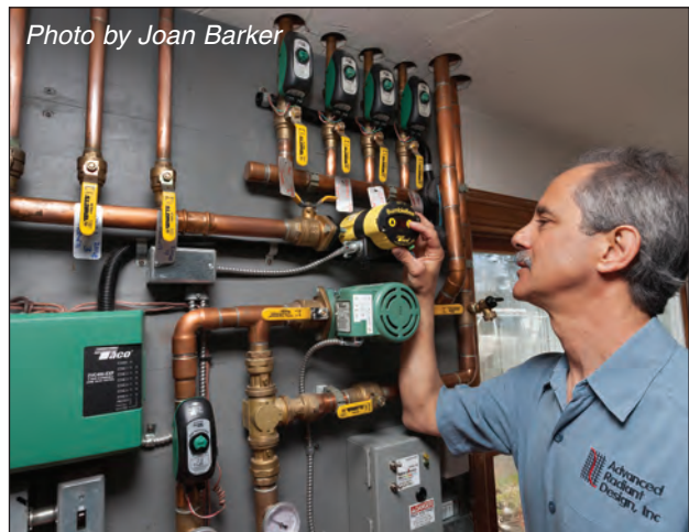
John Abularrage checks the function of a Taco Bumble Bee circulator at another biofuel job just a few miles down the road from the Triform facility.
